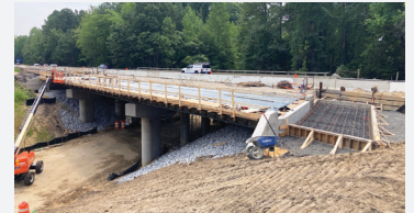
I-64 Gap Segment C Design-Build, James City County, VA
