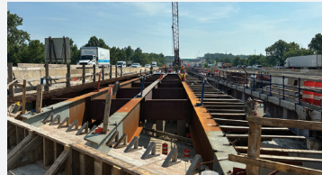
MD 24 Interchange, Harford County, MD
