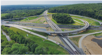
I-95 / SR 896 Interchange, Newark, DE
