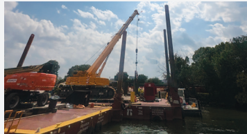
Long Bridge South Design-Build, Washington, D.C.
