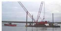
Route 52 Causeway Project - Ocean City, NJ
