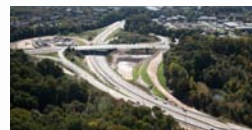
InterCounty Connector - Contract A - Maryland
